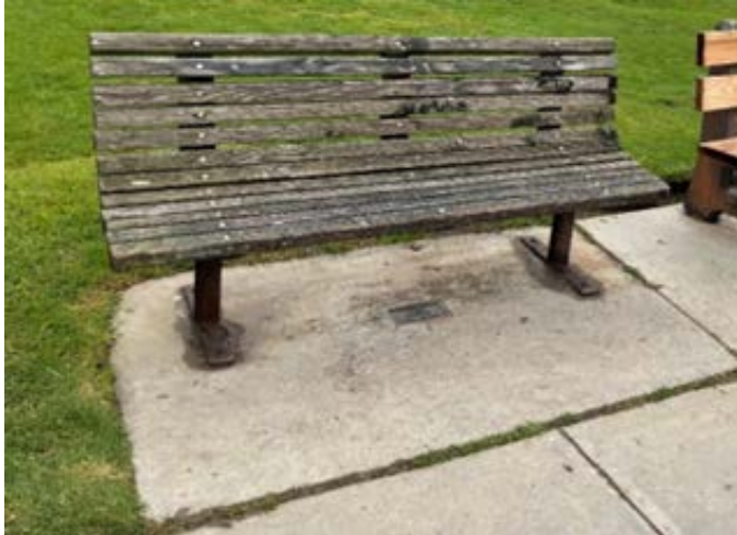
Old bench at Calumet Park with cracked and rusted metal supports and deteriorating wooden slats.
