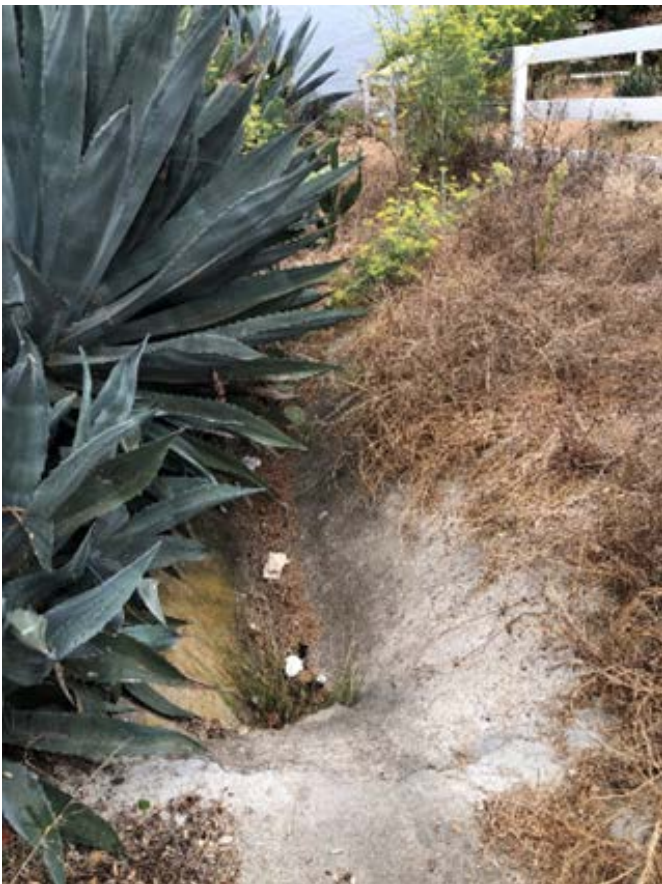
Right photo from 11/9/2022 after removal of debris and plants, repair of slope between culvert and the Park, and addition of a new concrete section towards the bluff edge.
