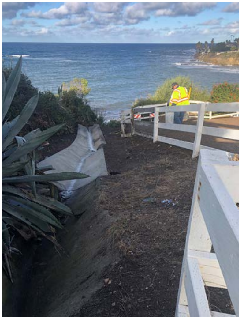
Right photo from 11/9/2022 after removal of debris and plants, repair of slope between culvert and the Park, and addition of a new concrete section towards the bluff edge.
